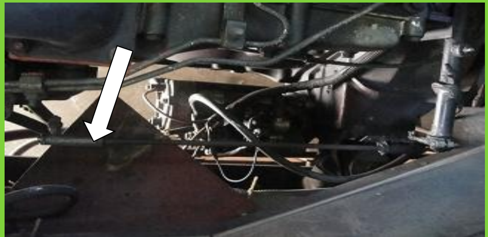
OPEN POSITION TO REPAIR ACCESS
